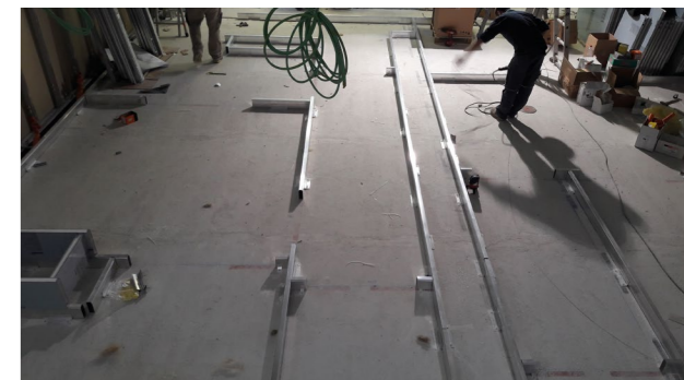
Fissaggio guide a pavimento Fixing rails to the floor Fixation des lisses au sol
